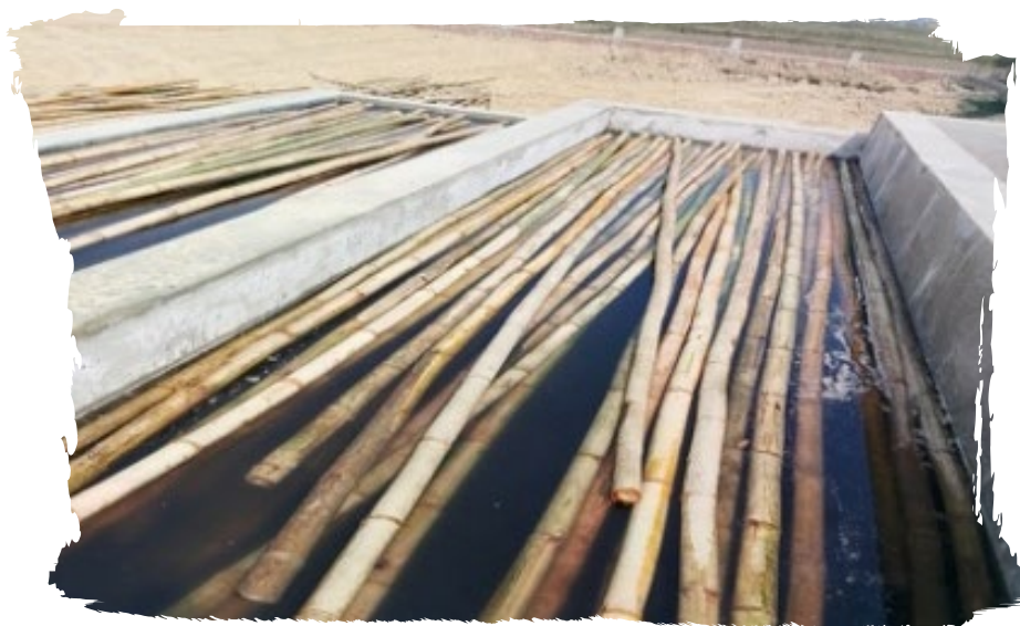
Community Improvement Center's bamboo treatment plant.
